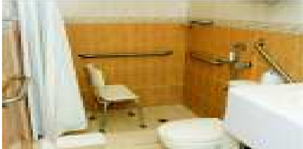
Figure 6.21 Bathroom with grab bars and plastic chair
